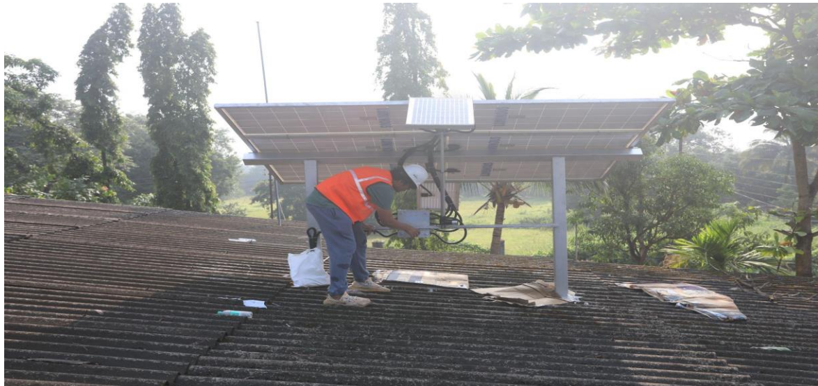
Image -2: Photo clicked during the installation of single-axis solar tracking system
