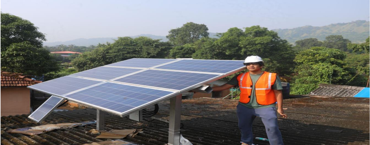
Image -4: Photo clicked after the installation of single-axis solar tracking system
