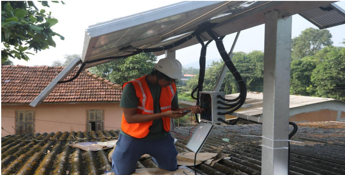
Image -1: Photo clicked during the installation of busbar box
