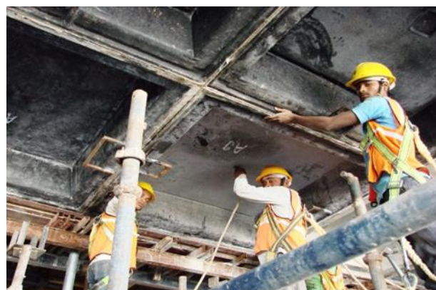
Fig 8: Removing moulds with the help of an air compressor
