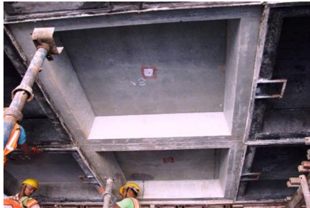
Fig 10: Aesthetic view of coffer slab
