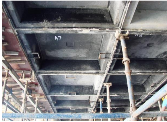
Fig 9: Shuttering of coffer slab
