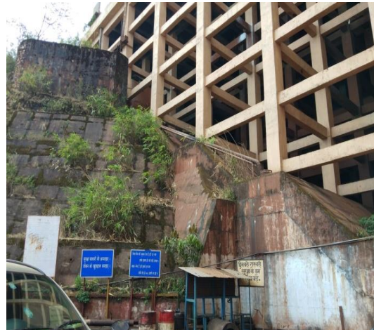
Fig. 3: view of Blanket wall at primary crusher entry.
