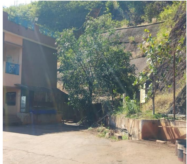
Fig. 6: NMDC Project office, Protection Works.
