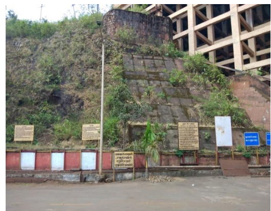
Fig. 1: Front view of Blanket wall
